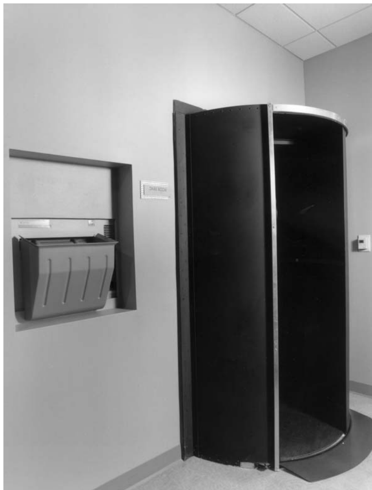
Figure 5-29. View of tech work corridor showing through-the-wall film processor (“daylight” side) and revolving darkroom door. (Design: Jain Malkin Inc.; Photographer: Glenn Cormier.)
