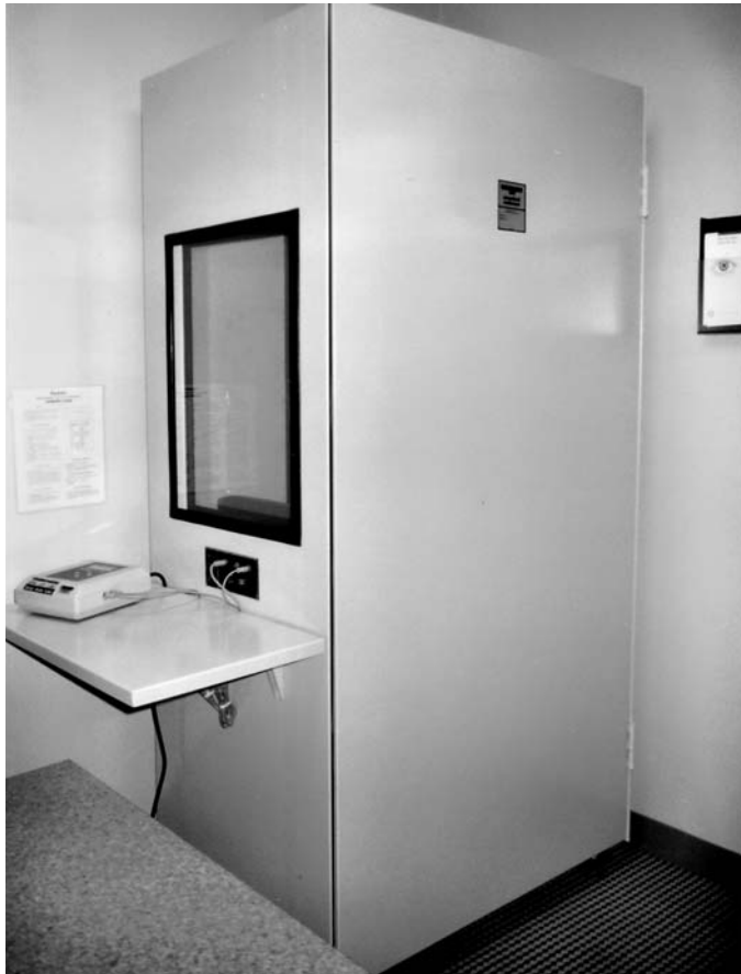
Figure 4-63. Prefabricated audio booth for testing hearing. (Photographer: Jain Malkin.)
