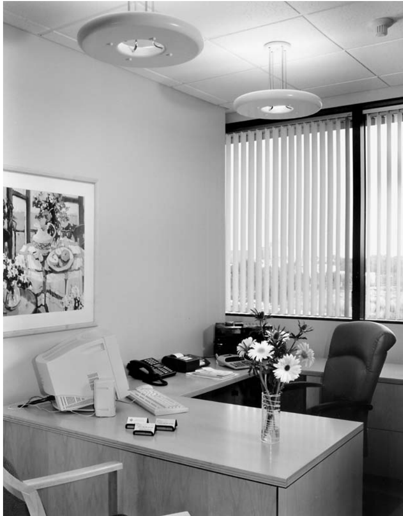
Figure 13-9. Fluorescent pendant lights in clinic administrator's office provide indirect light that bounces off ceiling and eliminates glare on CRT. (Design: Jain Malkin Inc.; Photographer: Glenn Cormier.)
