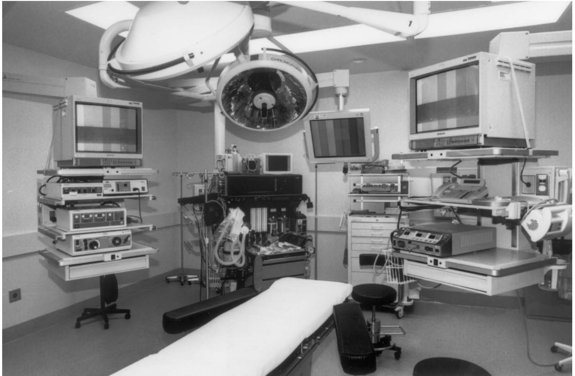
Figure 7-20. State-of-the-art laparoscopic operating room equipped with video-laparoscopic surgery “towers” suspended from the ceiling by power booms (articulating arms) to keep floor clear of clutter. (Photo courtesy: Hackensack University Medical Center, Hackensack, NJ)
