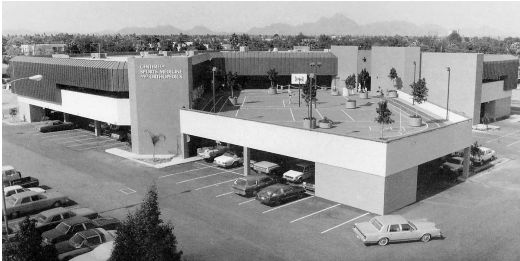
Figure 8-10. Center for Sports Medicine and Orthopedics, Phoenix, AZ. (Architecture: Devenney Group, Ltd., Phoenix, AZ; Photographer: Michael Much.)
