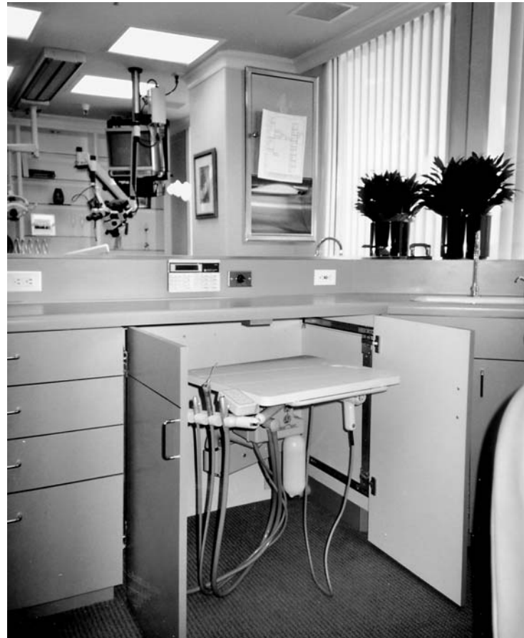
Figure 10-34. Custom casework in treatment room features retractable doors to conceal assistant's mobile cart. (Photo courtesy: Cheryl Sheets, D.D.S.; Photographer: Jain Malkin.)
