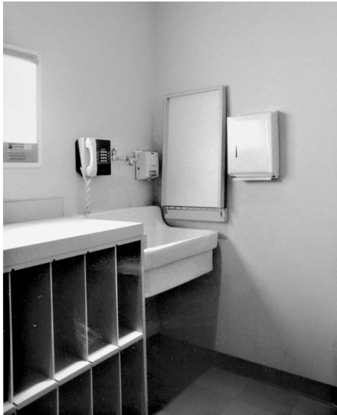
Figure 5-18. Tech work area, sorting and viewing counter. Note sink under hinged countertop. (Design: Jain Malkin Inc.; Photographer: John Christian.)
