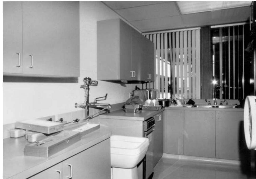
Figure 7-24. Soiled workroom with clinic service “flush” sink and sterilizer. (Design: Jain Malkin Inc.; Photographer: Jain Malkin.)
