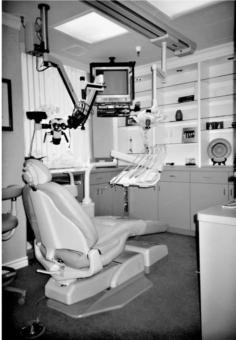
Figure 10-13. This treatment room has a ceiling-mounted operating microscope and TV monitor as well as centrally piped medical gases (note faceplates at toe of chair, left side). Glass shelves in front of patient display art objects. (Photo courtesy: Cheryl Sheets, D.D.S.; Photographer: Jain Malkin.)
