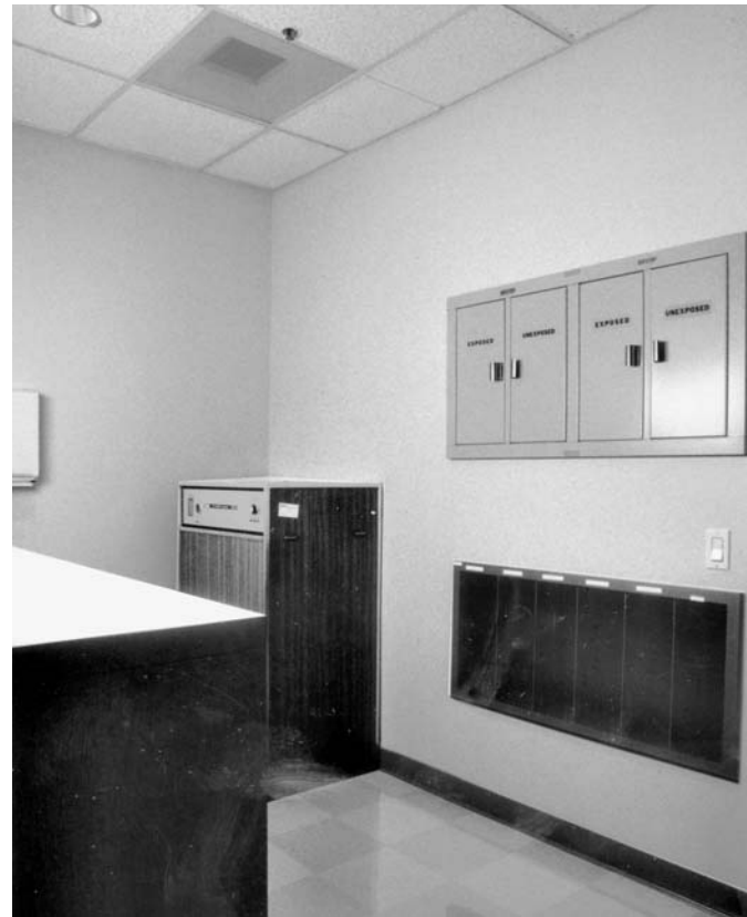
Figure 5-19. Tech work area (opposite side). Note pass boxes to darkroom and automatic processor (outdated model) and film sorting bins under pass boxes.
