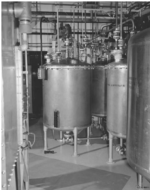
Figure 11.46 Image of the Los Alamos mixing vessel.
