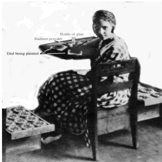
Figure 6.2 Close-up of the workshop, this one in Ottawa, Illinois. 3
