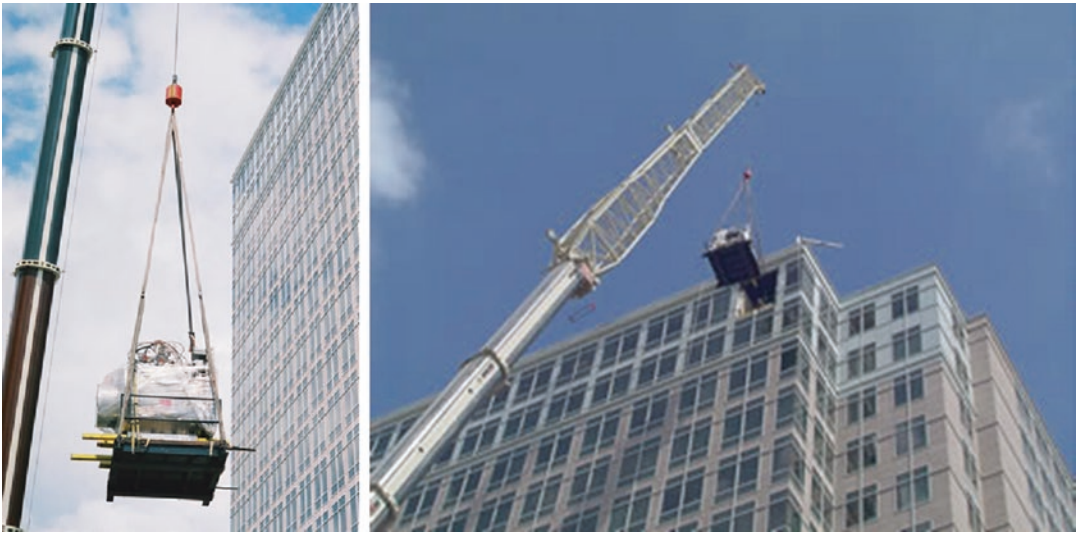
Fig. 1 These photos were taken during the installation of an MRI scanner at Resurgens Orthopaedics in Atlanta, GA on the 19th floor of their Crawford facility. Courtesy of Resurgens Orthopaedics, Atlanta, GA
