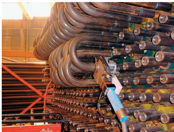
Figure 5-82 Photo of scanner clamped onto boiler tubes during construction inspection.
