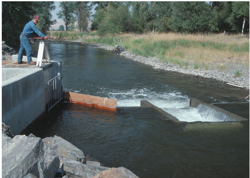
Fig. 11.4 Irrigation turnout upstream from dam in stream
