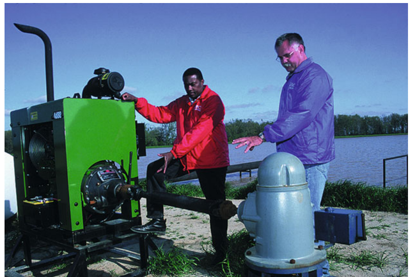
Fig. 9.2 Centrifugal pump and motor (Wikipedia)
