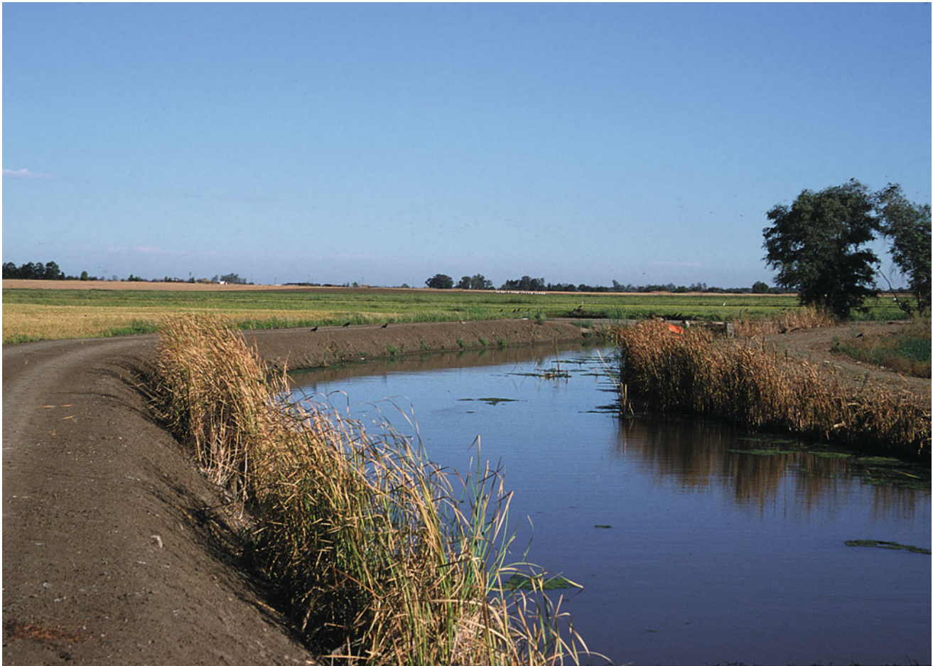
Fig. 11.7 Tailwater recovery channel (Credit NRCS Jeff Vanuga)
