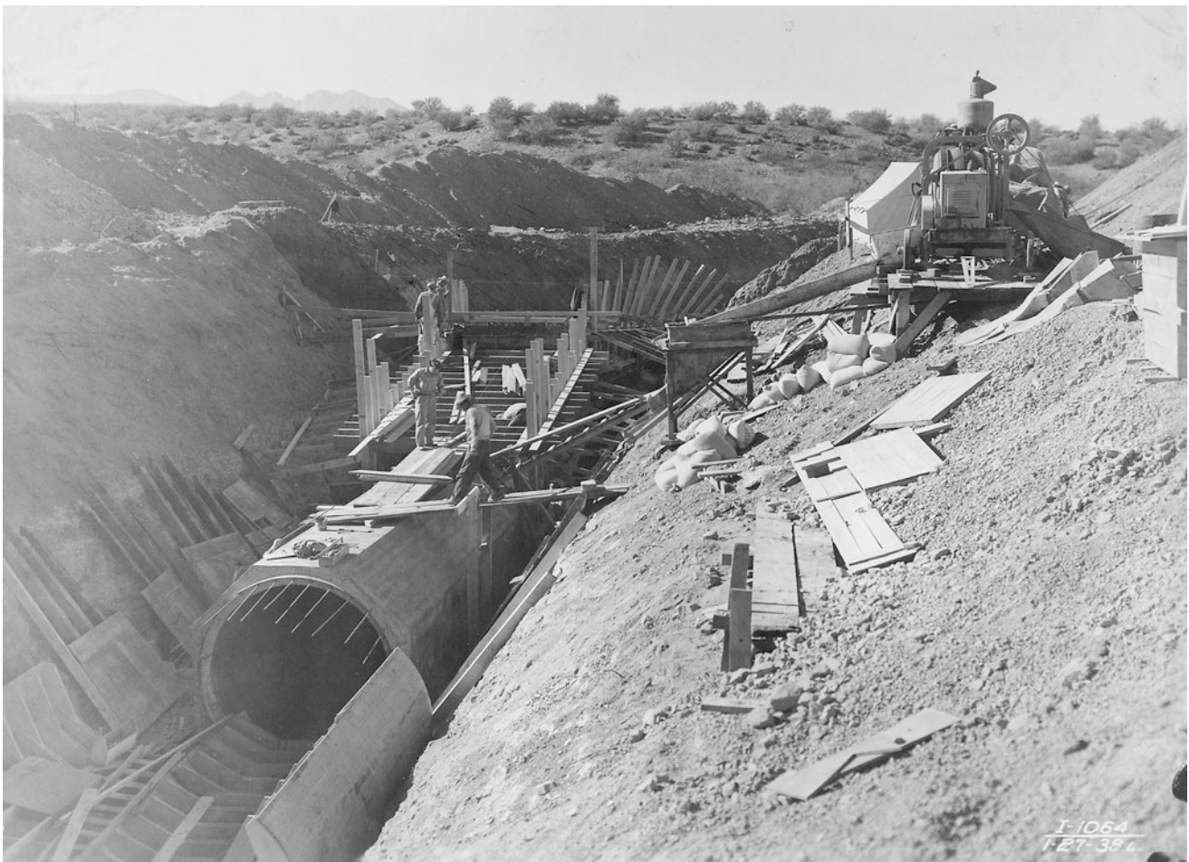
Fig. 11.11 Partially completed concrete siphon on Salt River Project (Credit USBR)
