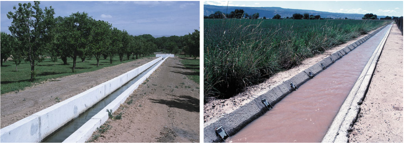
Fig. 11.1 Square and trapezoidal irrigation ditches (Credit NRCS)
