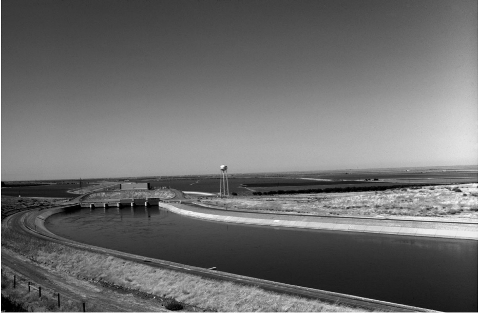
Figure 13.7 The California Aqueduct takes ‘blue water’ from the Sierra Nevada in the north of the state and delivers it to fruit farmers and other producers in the Central Valley and beyond (MKVC).
