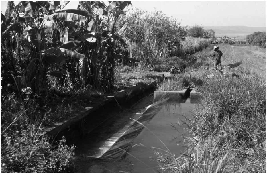
Figure 13.6 Water for irrigation is delivered to individual small farms from a diversion weir on a river through a network of small canals and control structures – Swaziland (MKVC).
