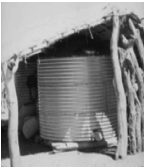
Fig. 5.26 Metal grain storage bin.
