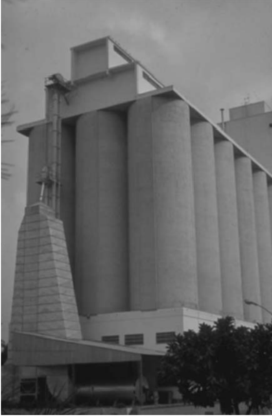
Fig. 5.31 Large round silo complex.
