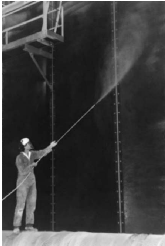
Fig. 6.22 Diatomaceous earth slurry spray application.
