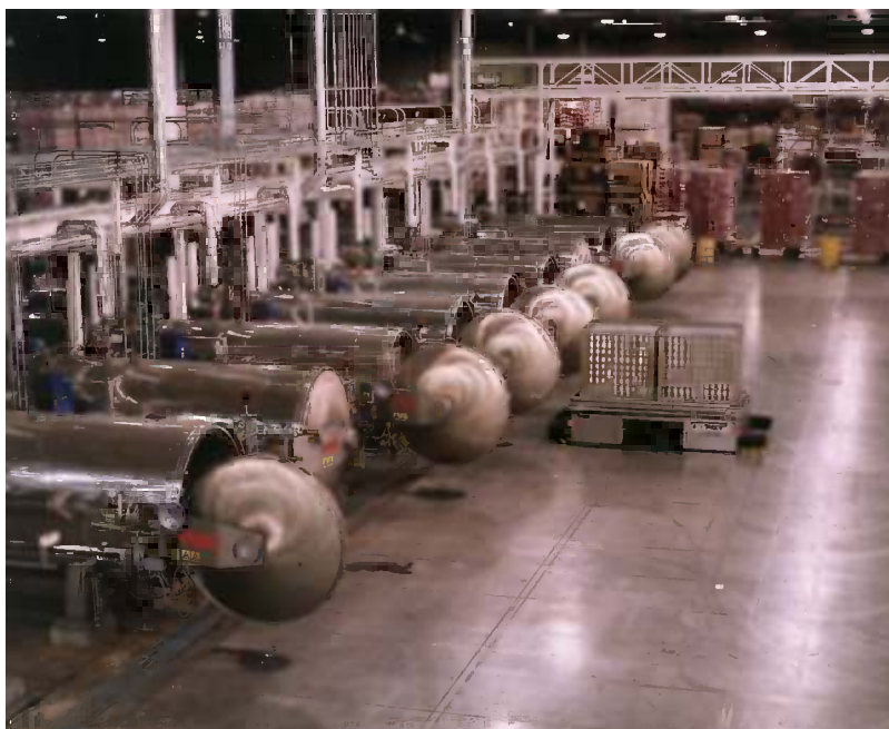
Figure 17.19 Modern cook room showing battery of retorts arranged for automated loading and unloading. (Photo courtesy of JBT FoodTech, formerly FMC FoodTech, Madera, CA)
