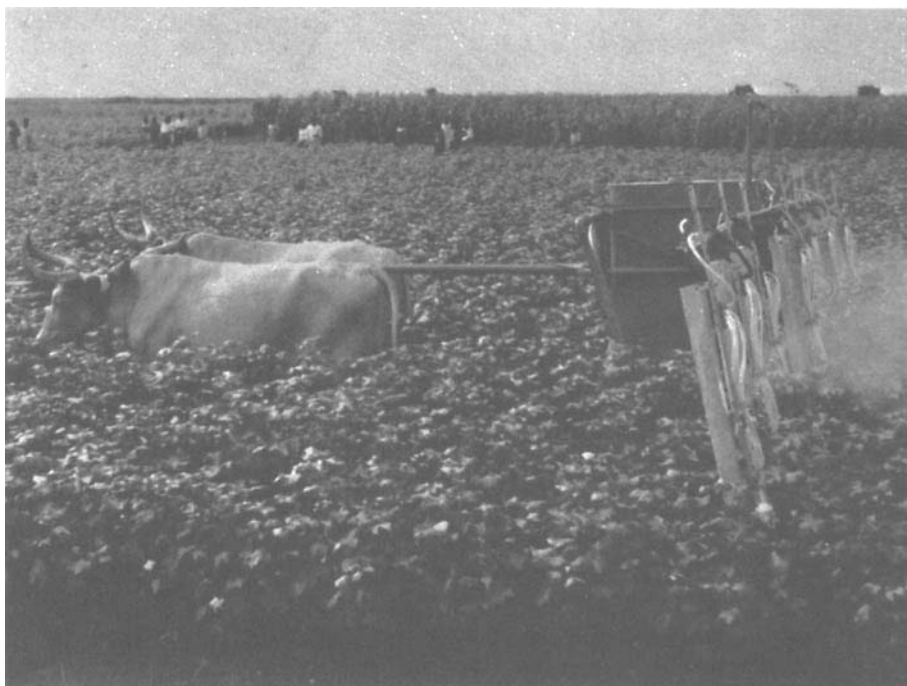
Fig. 7.24 Animal-drawn sprayer with engine-driven pump.
