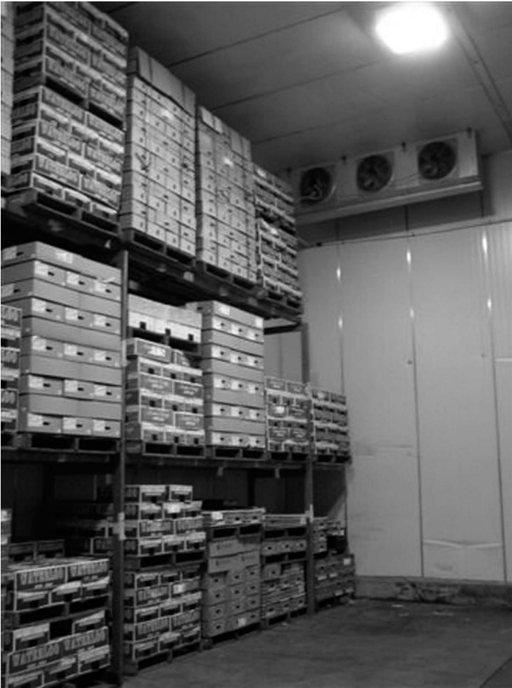
Figure 7.4 A cool room in which the air is blown through the coils by fans mounted at the back of the coils ( forced draft cooling ). The more common arrangement is to mount the fans in front of the coils ( induced draft cooling ), which gives better air distribution. In this example, the palletised produce is placed on racks.
