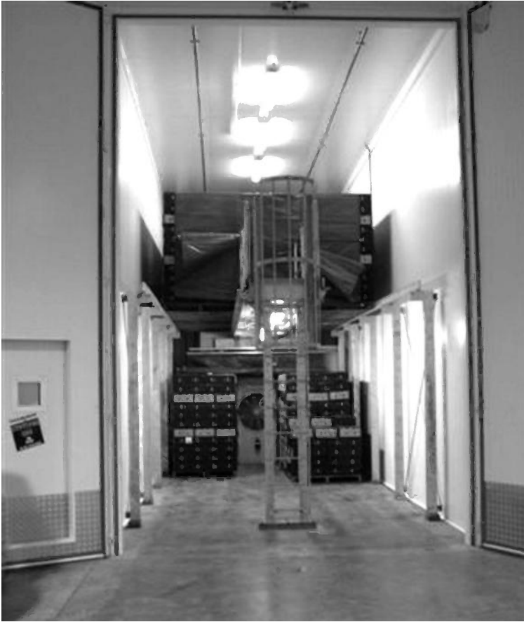
Figure 11.3 A modern double-deck controlled ripening room for bananas using forced-air circulation. The boxes are vented to allow air to be drawn through the packed fruit.
