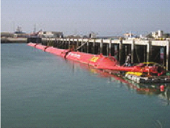
Fig. 13.6 Ocean Wave Power engines in the harbour of Peniche/Portugal
