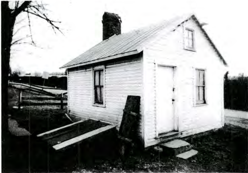
The entrance to the Whites' fine old stone-walled root cellar is under the bulkhead on the side of this summer-kitchen building.
