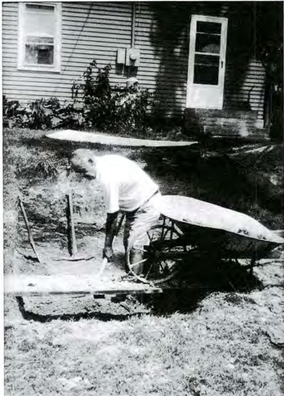
Digging out the Harper root cellar.
