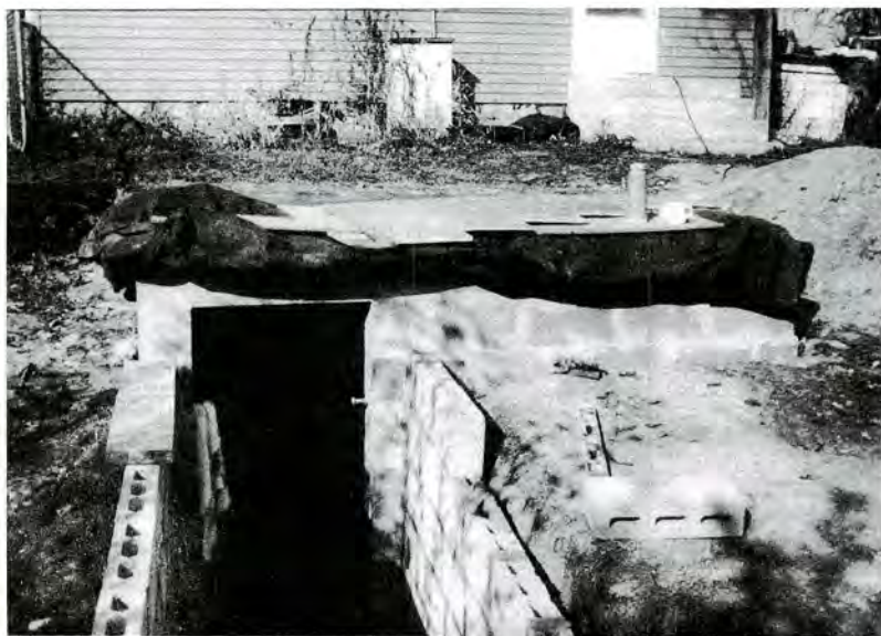
The Harper root cellar during construction.
