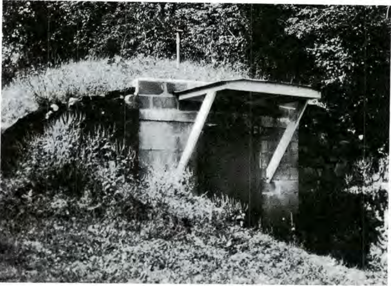
The Senft root cellar is dug into a hill and has an awning to protect the doorway from sun and rain. Note that the stone facings on the sides of the hill surround the root cellar.
