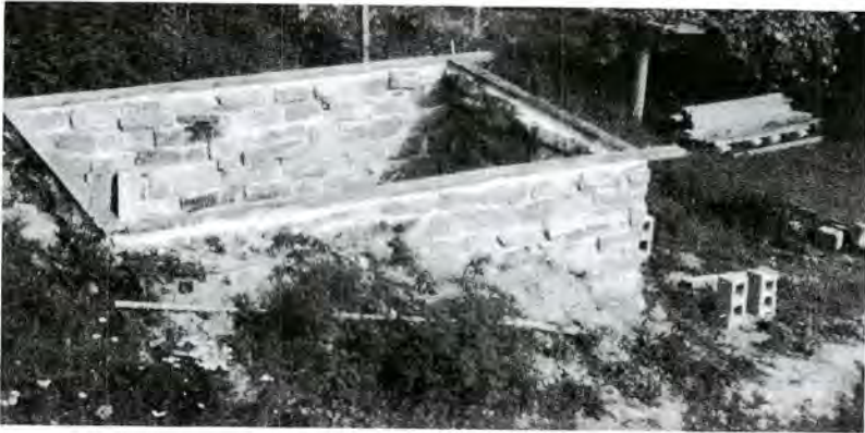
The Woolings’ root cellar—ready for the roof.
