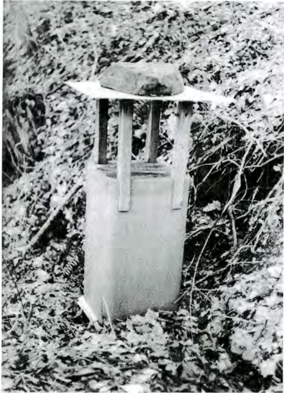
A terra cotta flue liner serves as the vent pipe for the Knier root cellar.
