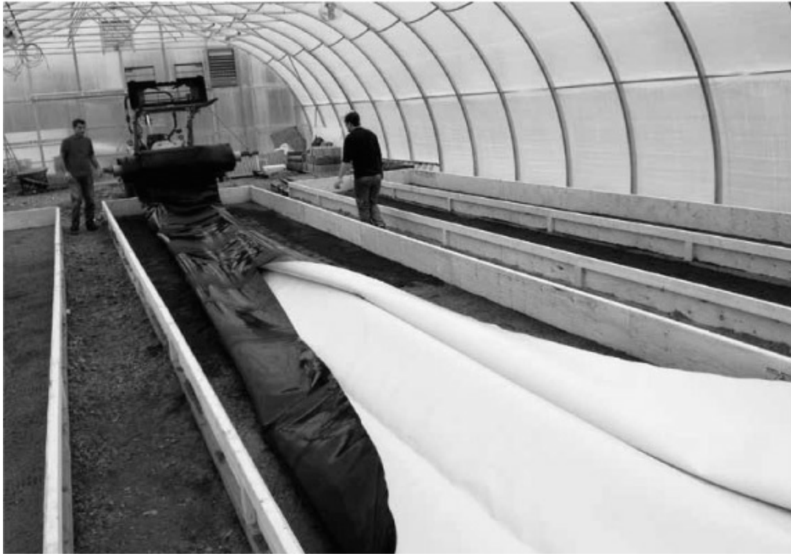
Rolling out the LDPE for liner installation.
