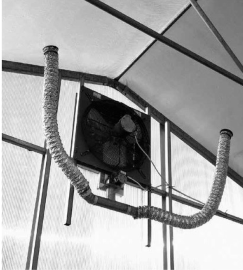
Peak vent and double-layer poly inflation blower.
