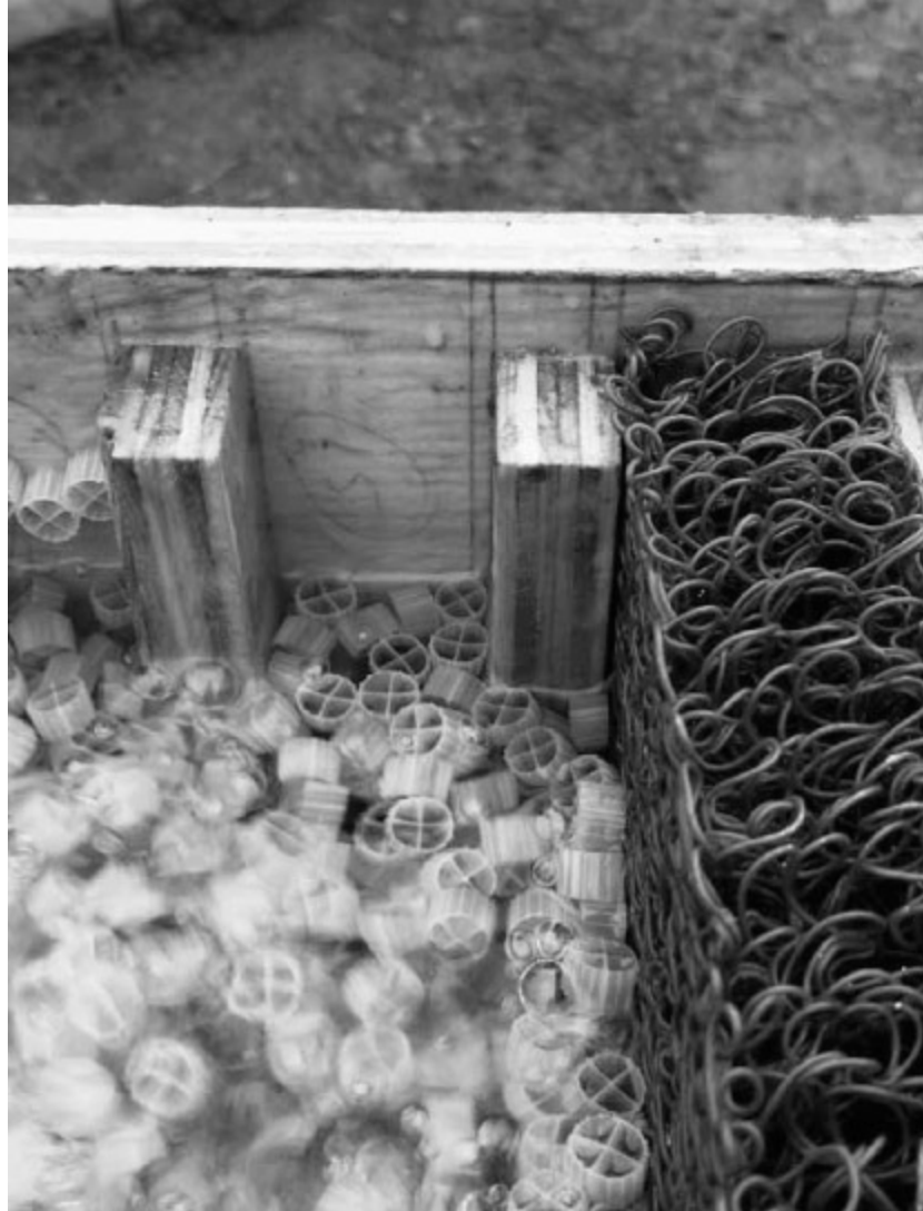
Filter screen (right) and MBBR media (left) in the CFB.
