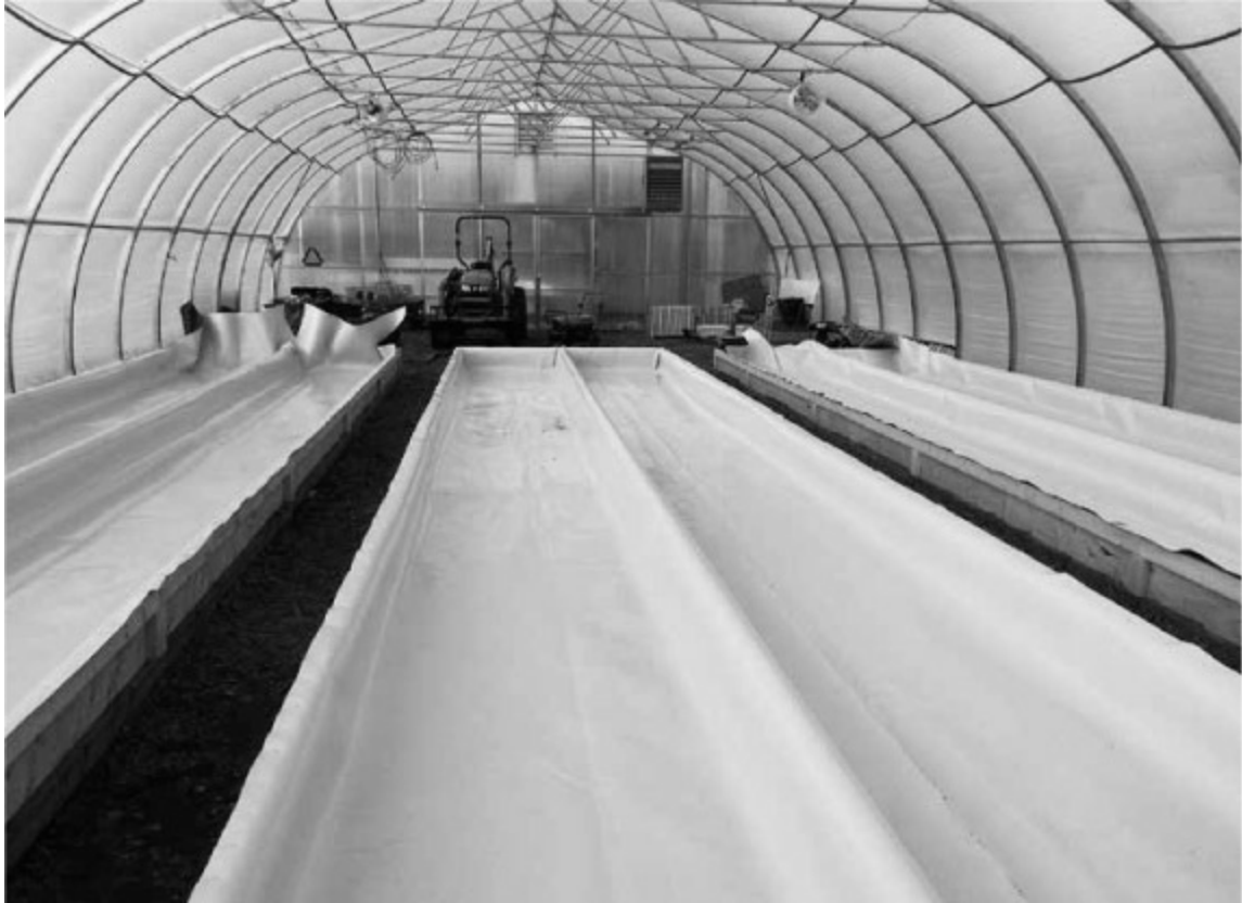
Nearly completed trough liner installation.
