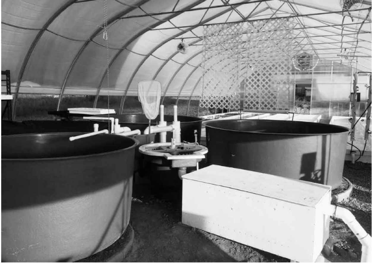
The fish tanks, Tank Manifold and filtration systems (RFS and CFB) at our farm.
