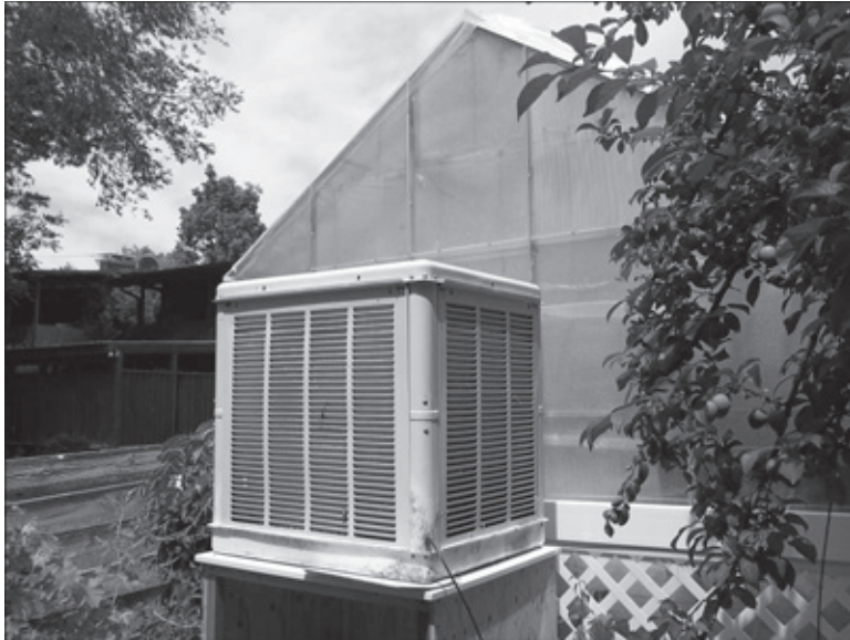
This aquaponics gardener has installed a used swamp cooler in the greenhouse. Swamp coolers work well in dry climates.
