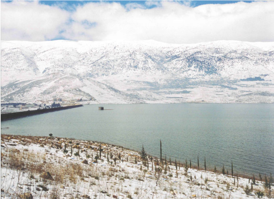
Fig. 2.1 Dam side of the Qaraaoun Reservoir as observed in winter 2017
