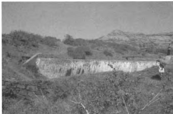
Fig.R.3: Check dams act as water reservoirs, where water can be used for irrigation purpose. Courtesy: Dr. Vrishali Deosthali, Department of Geology, University of Pune, India.
