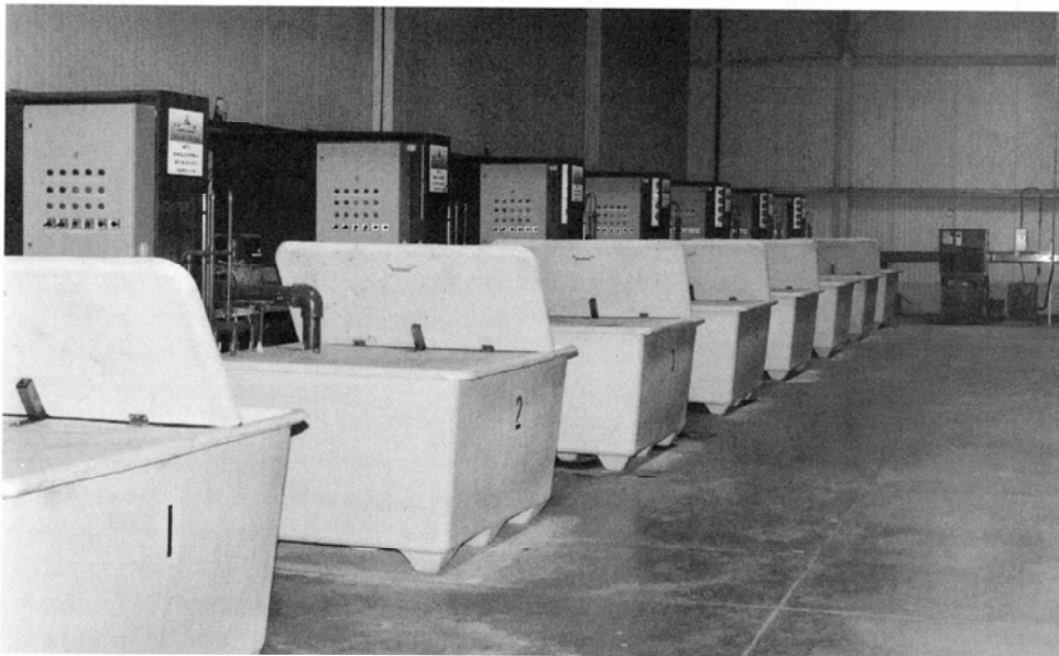
Commercial nutrient mixing and delivery systems.
