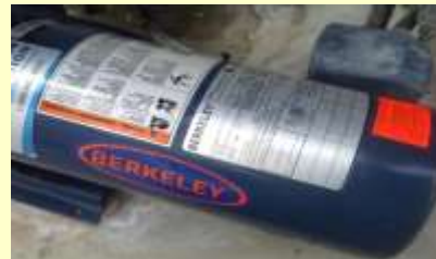
Low pressure water pump (1 HP).
