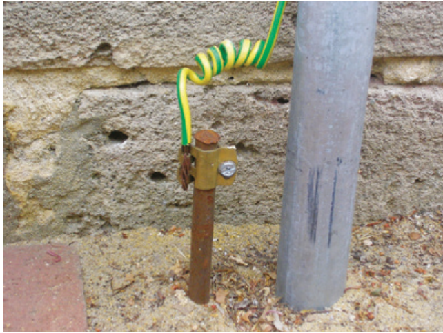
Fig. 16.2 Wire connected to the earth
