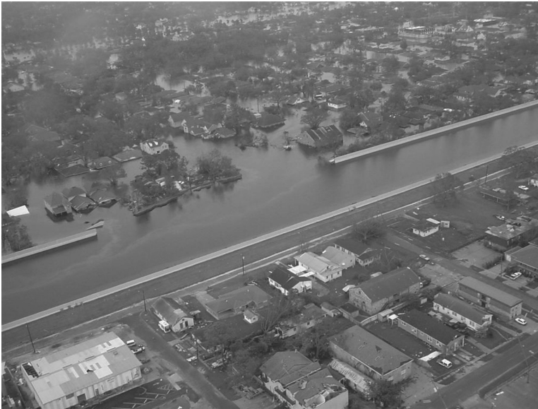
(b) Breached Floodwall
