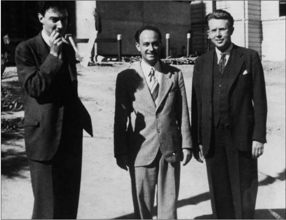
LEFT TO RIGHT: Oppenheimer, Fermi, E. O. Lawrence at the construction site for the Berkeley accelerator, 1939.
