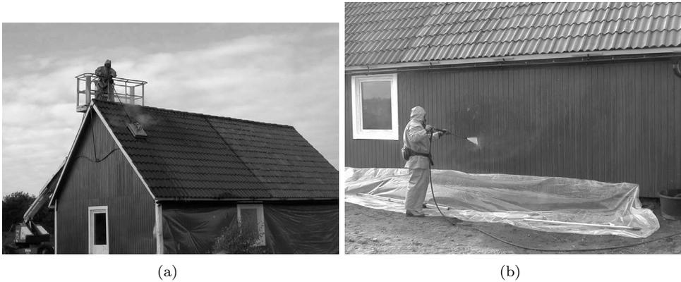
FIGURE 7.47 Decontamination of a building using wet padding of external contamination on the roof (a), and subsequent high-pressure washing to remove the suspended radionuclides (b). Note that the radionuclides washed off from the roof must be collected on the ground and treated as radioactive waste.
