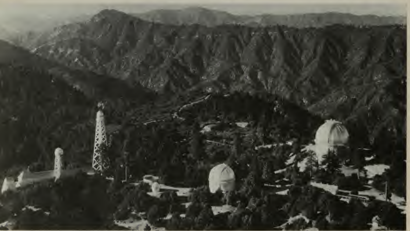
Buildings and instruments of modern observatories. Top: the 200-inch telescope and its dome on Mt. Palomar. Bottom: the complex of buildings on Mt. Wilson.
