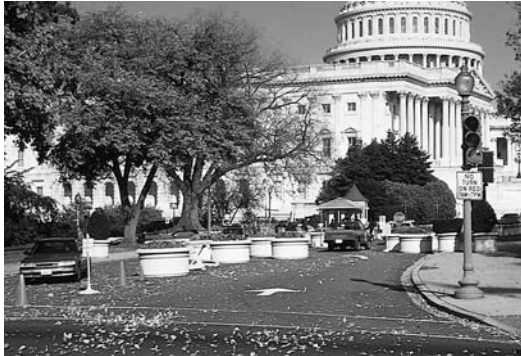
FIGURE 24.2 Vehicle Barriers (Planters); U.S. Capitol Grounds.
