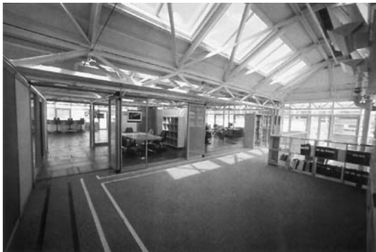
FIGURE 12.16 In the Robert L. Preger Intelligent Workplace, 75% of the Facade Area is Glazed with High-Visibility, Low Shading Coefficient Glass, Maximizing Effective Daylighting throughout the Year. The Windows Are Operable To Allow Natural Ventilation Cooling for 9 Months and Water “Mullions” Dissipate Waste Heat for Energy Efficient Perimeter Heating. (Architects Bohlin Cywinski & Jackson, Pierre Zoelly, & the CMU Center for Building Performance.)
