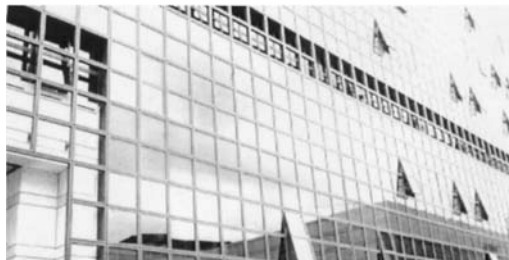
FIGURE 12.10 In the Ministry of Finance in Paris, Operable Windows Provide Occupants with Outside Air As Desired, but Avoid Energy Waste by Shutting Off the Perimeter Heating/Cooling Unit (ABSIC; France, 1991).
