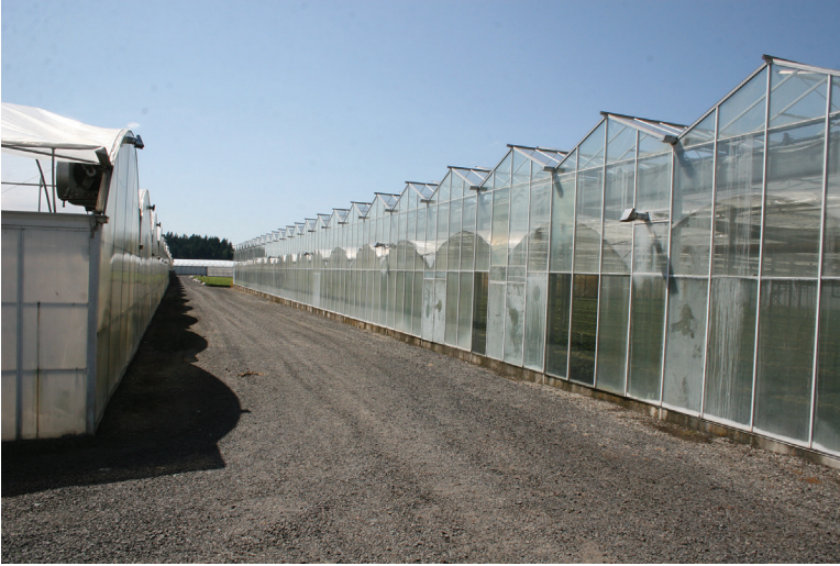
Figure 1.1 Glass greenhouse structures.
