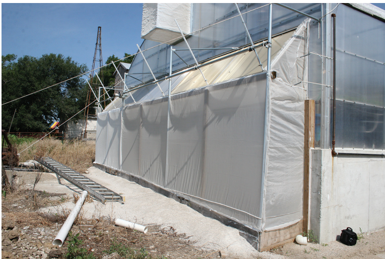
Figure 5.4 Installation of insect screening on south side of greenhouse.
