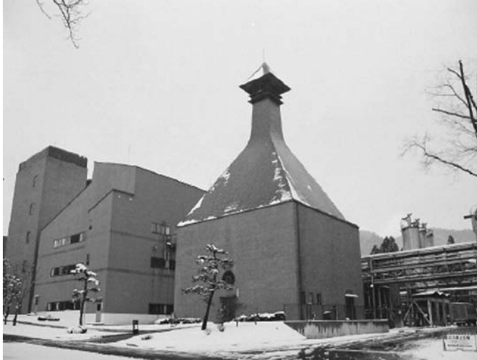
Figure 21.1 Drying kiln, with its unique chimney.
