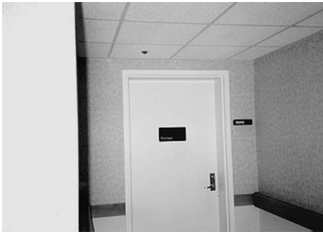
FIGURE 7.11 Door to isolated back store room.
