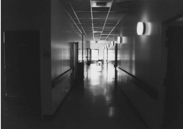
FIGURE 9.36 Labyrinth effect produced by the existing building and the similarity of the corridors.
