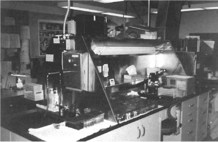
FIGURE 28.2 Workstation for toluene and alcohol procedures and storage with slot-type local exhaust ventilation at Jewish General Hospital. Slot air exhaust is located at the back of the hood.
