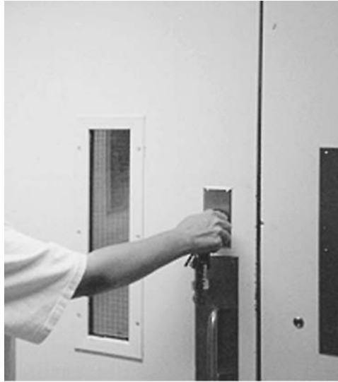
FIGURE 7.7 Skeleton key locks require workers to “remember” to manually lock them.
