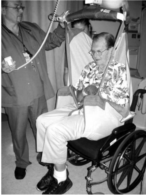
Ceiling-mounted patient lifts
