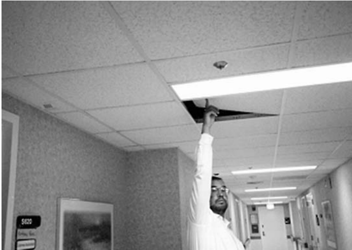
FIGURE 7.9 Tiles are easily removed for hiding contraband.
