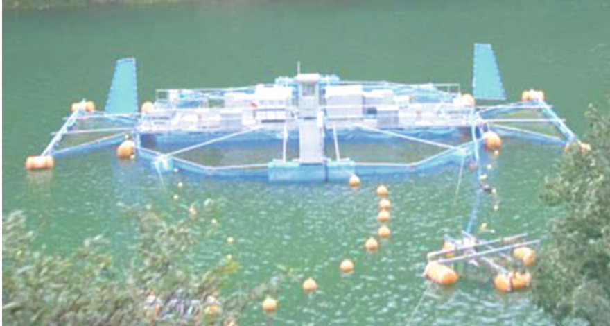
Fig. 6.8 A large-sized algae treatment system in 2006
