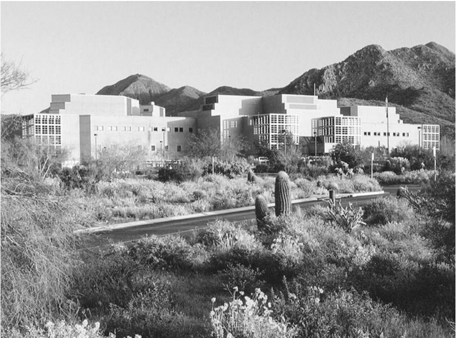
Mayo Clinic Building, a five-story outpatient facility located on the Scottsdale campus, has 240 exam rooms, outpatient surgery, endoscopy, laboratory, radiology, pharmacy, and multilevel underground parking.
