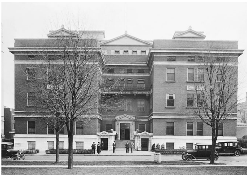
1914 Mayo Clinic building, the first building ever designed to accommodate an integrated, multispecialty group practice of medicine.
