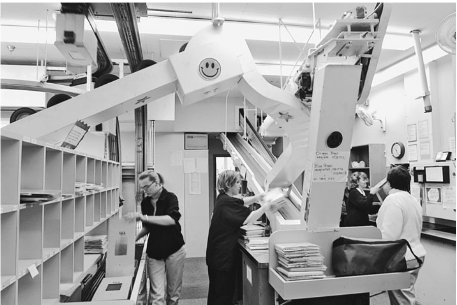
Lifts and chutes in the Mayo Building's medical record distribution center were rendered obsolete by the electronic medical record early in the twenty-first century.
