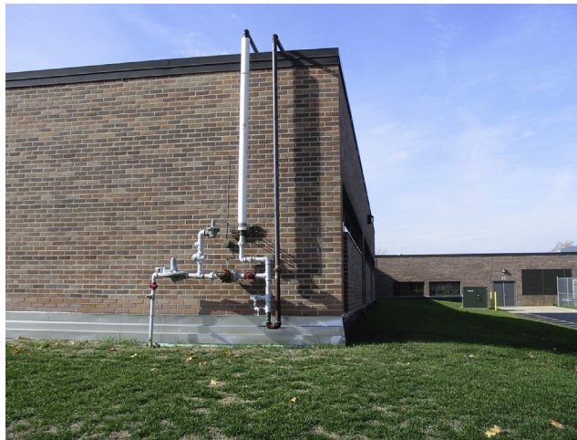
FIGURE 4.8 Roof Access Before.
