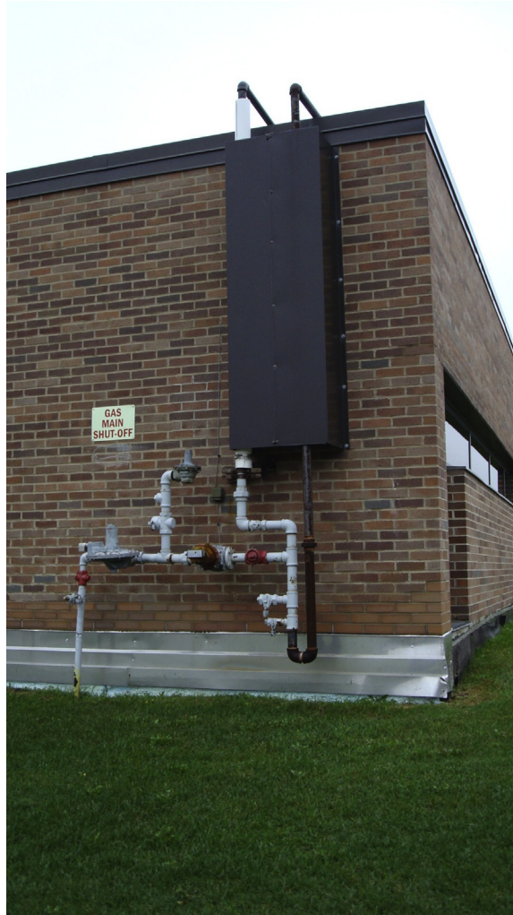
FIGURE 4.9 Roof Access After.
