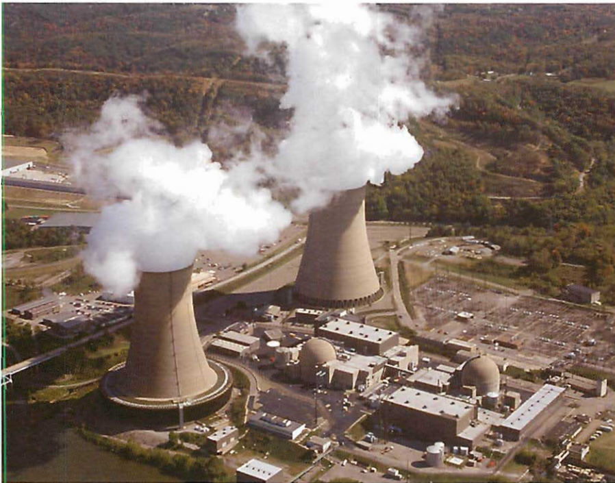
Figure 5.14 The Beaver Valley Nuclear Power Station in Pennsylvania. The two nuclear reactors are in the two containment buildings with rounded roofs in the lower center and lower right. The large towers emitting steam provide cooling for the reactors. The rectangular buildings contain the electric generators. The steam comes from water taken from a nearby river; it does not come in contact with the nuclear fuel, and it is not made any more radioactive by the power plant. (Courtesy of U.S. Nuclear Regulatory Commission.)
