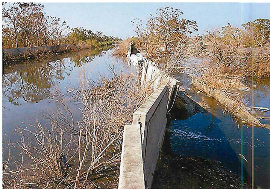
Figure 2.2 Levees in New Orleans, shortly after Hurricane Katrina, broken at their thermal expansion joints. They didn't break from heat, but from the pressure of the flood. However, the expansion joints were the weakest part of the levee. (Courtesy of U.S. Army Corps of Engineers.)
