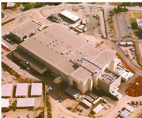
Figure 5.16 The National Ignition Facility (NIF) laser building at Livermore. The goal is to ignite thermonuclear fusion of tritium and deuterium using lasers to power the implosion. (Photo courtesy of U.S. Department of Energy.)
