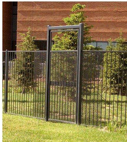
FIGURE 17-3 Example of a decorative iron fence providing a pleasing definition and security for an outside garden area. (Courtesy of The Children's Hospital, Aurora, Colorado).
