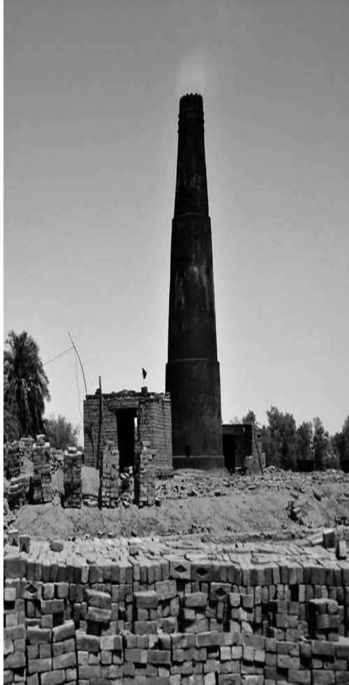
FIGURE 3.1 WHWB brick kiln study site in Nepal. (Photograph courtesy of Steve Thygerson.)
