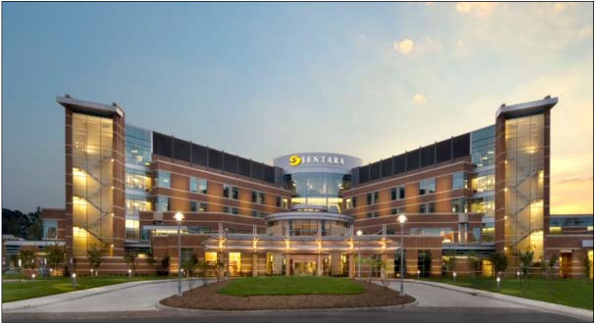
2.9 Sentara Williamsburg Regional Medical Center, Replacement Hospital in Williamsburg, Virginia. Photo © VanceFox.com
