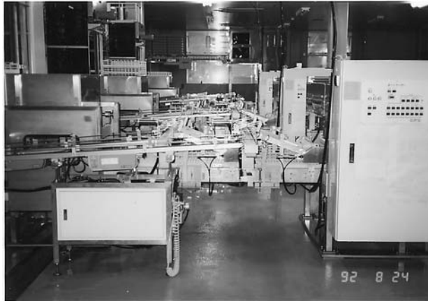
Figure 17 Automatic in-caser (slide system). (Courtesy of Suzuyo Kogyo Co. Ltd.)
