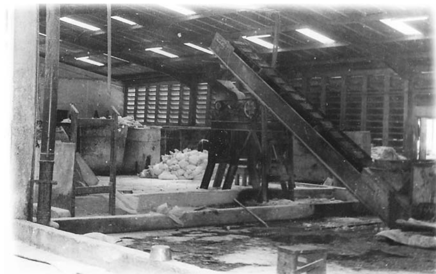
Figure 11 Commercial industrial gari production. Washed roots being elevated onto an electric pulper. (Courtesy of the Federal Institute of Industrial Research, Oshodi, Lagos, Nigeria.)
