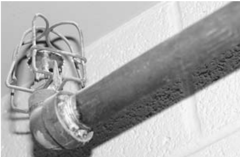
FIGURE 9.6 Sprinkler head
