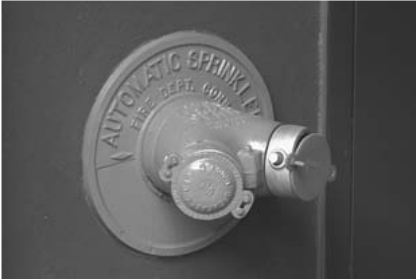
FIGURE 9.7 Sprinkler-system connection
