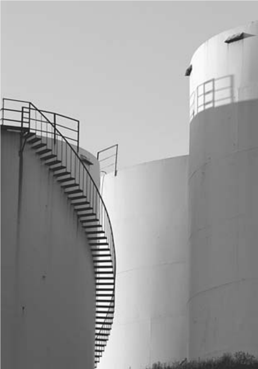
FIGURE 3.4 Outside aboveground storage tanks
