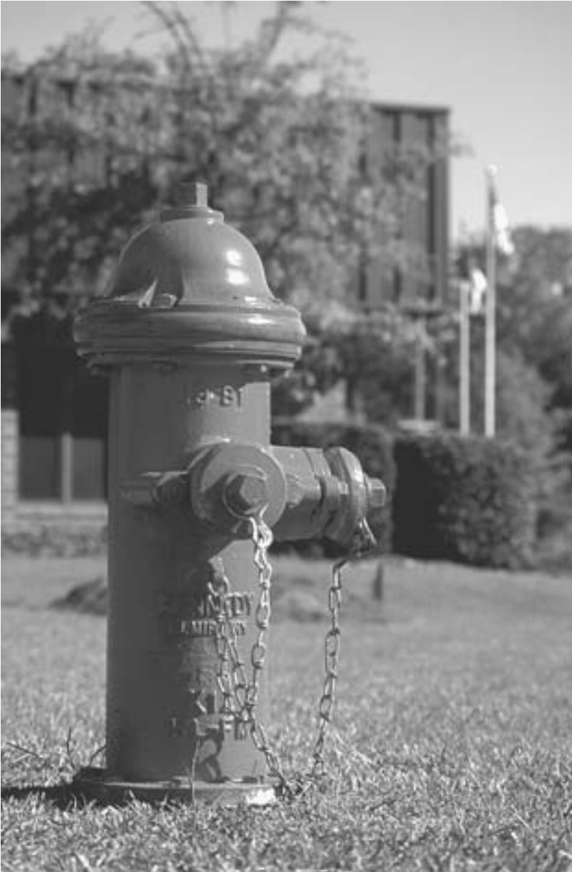
FIGURE 9.8 Barrel-type fire hydrant
