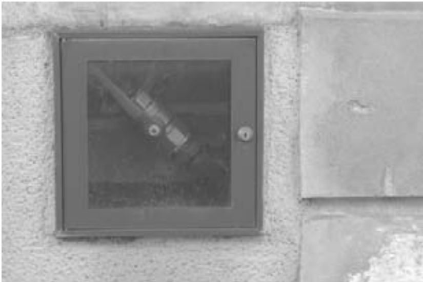
FIGURE 9.9 Standpipe hose case
