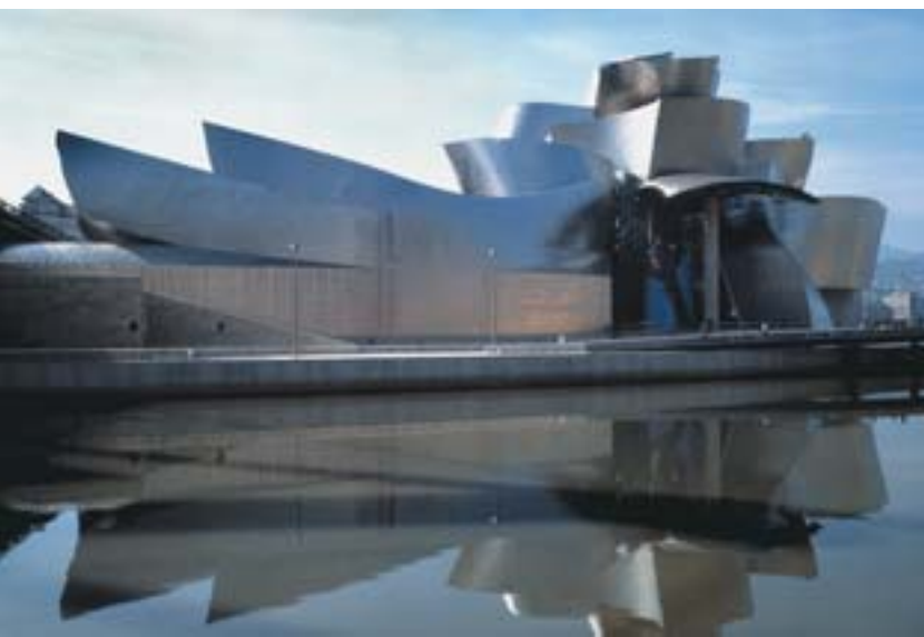
TITANIUM SHEATHES the Guggenheim Museum Bilbao in Spain. If the metal were cheaper, designers and engineers would use it more frequently.
